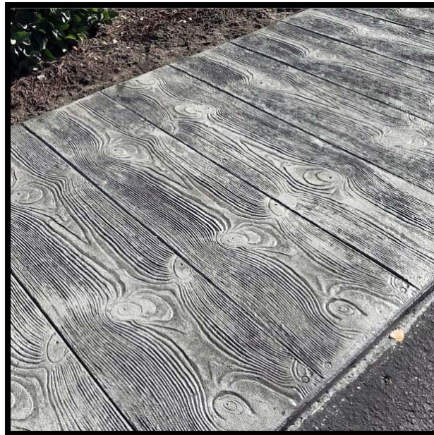
Figure 2 Wood Grain Stamped Concrete
