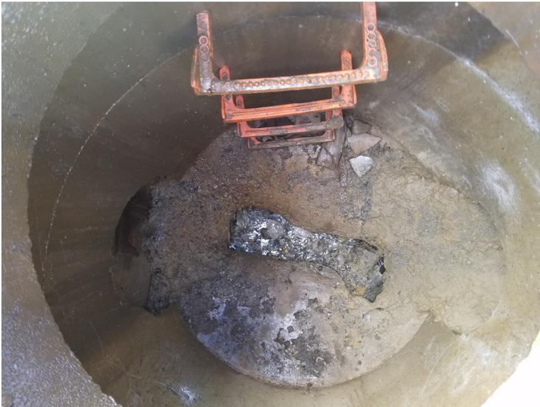
**Manhole with bottom covered in debris.** Manhole that appears it was not completed when installed has mud and debris covering the bottom and partially blocking the troughs. Sewer mapping shows 3 pipes at this location.
