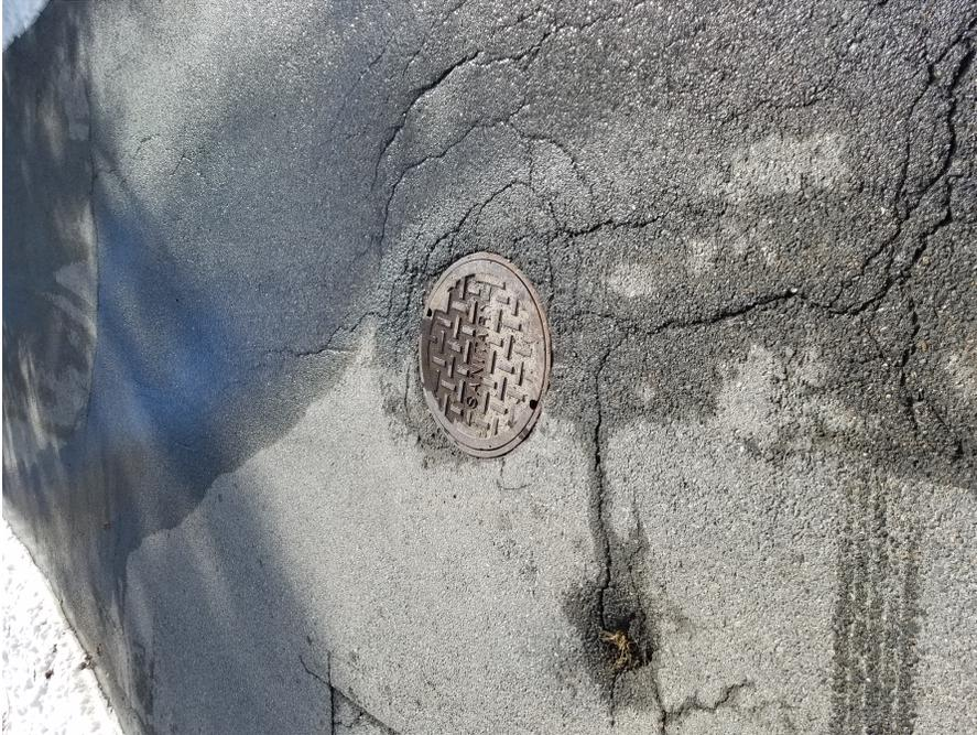
**Manhole Cover @ Davis and North Streets.** Pavement Cracking and settling around the structure and a small sink hole at the bottom center of the photo.
