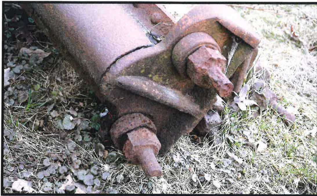
End view of bridge seat and corroded threads from lower tension straps.
