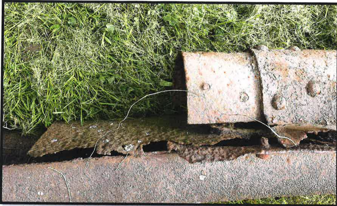
Splice coupling - note coupling riveted to one end of tube in shop and bolted through drilled and tapped hole on adjacent tube section in the field. Note also that plate has completely corroded between the flange of the top and bottom tube sections. Image from arch #6.
