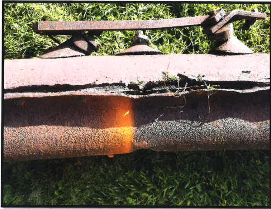
Rust bulge, rivets popped, Arch 1 joint U3, note missing portion of cruciform vertical
