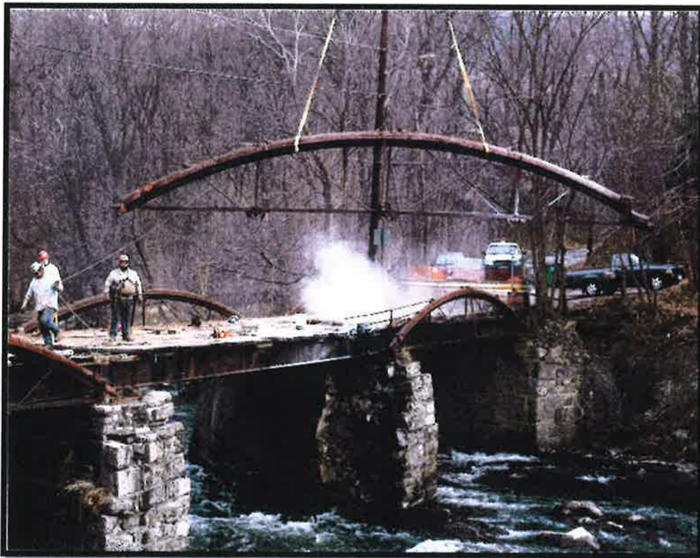
Removing Center Arch
