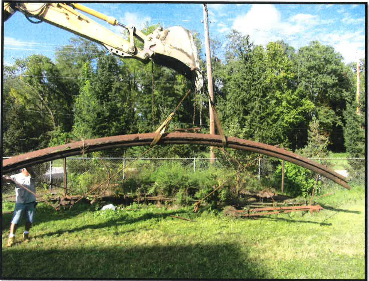
Lifting first arch from pile
