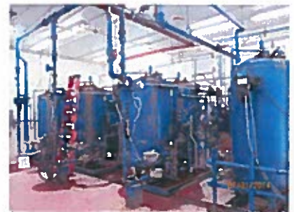
Still Pond Water Treatment Plant Existing pressure Media Filter Systems
