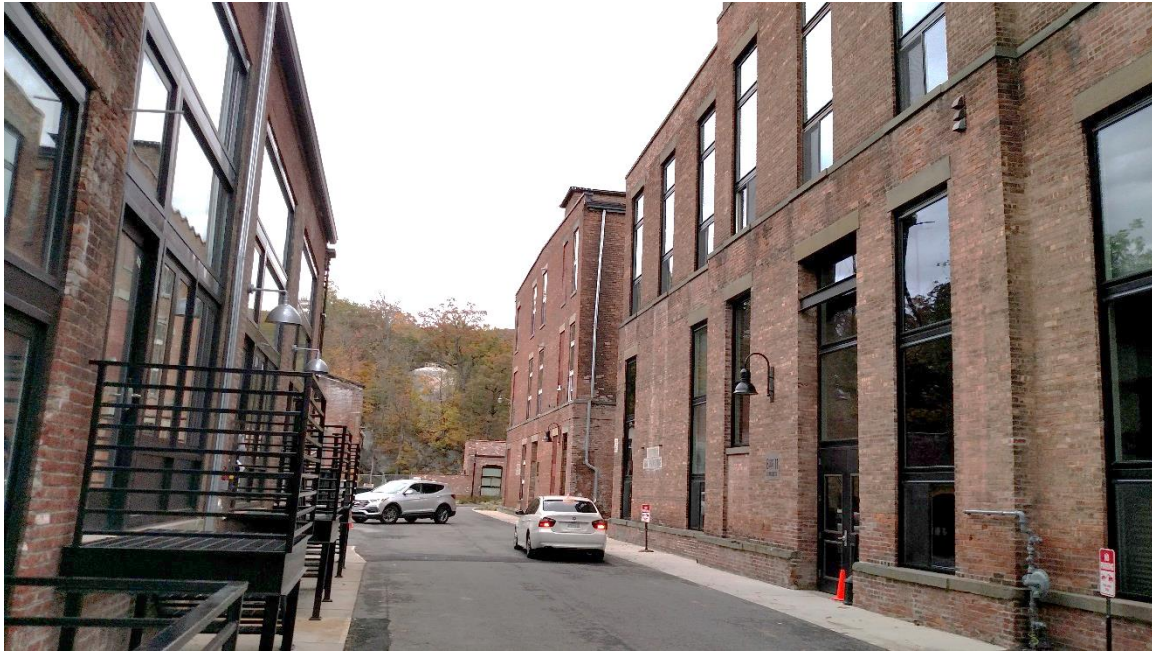
Photo 9: View to the northwest from the hydroelectric facility along Mason Circle between Building 11 (left) and Buildings 1-4 and 19-20 (right).
