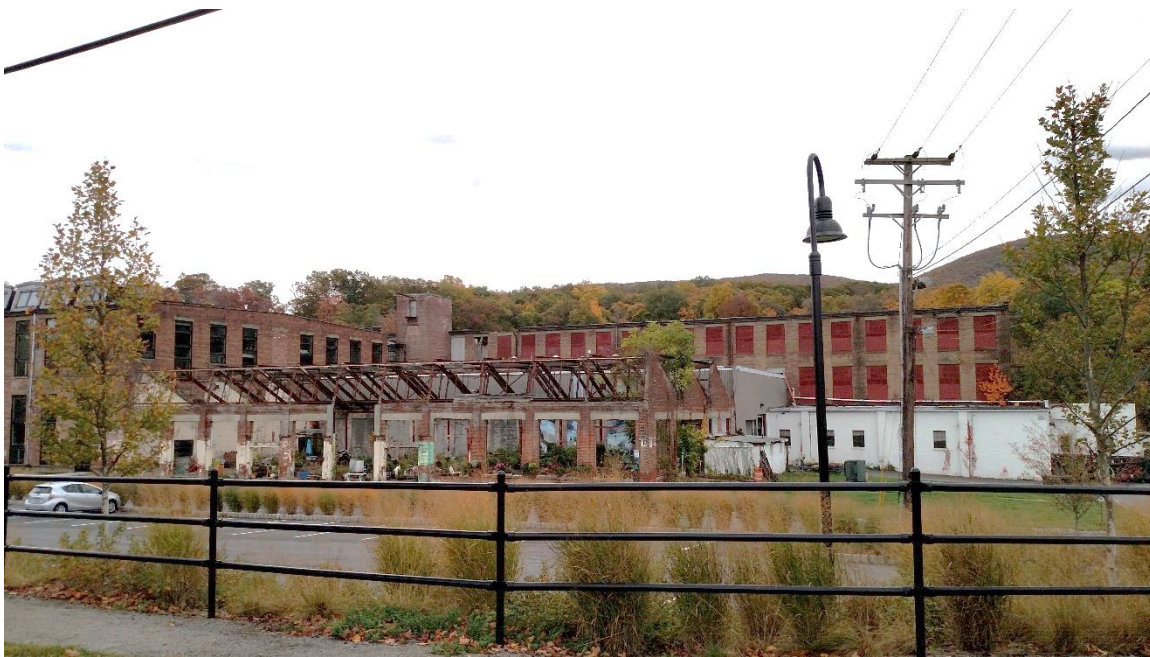
Photo 12: View to the southeast across the historic complex from Front Street.
