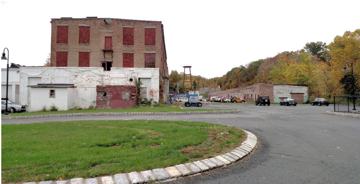
Photo 11: View to the northeast of Building 16 (left) and Building 9 (right) within the Proposed Site plan Amendment area.
