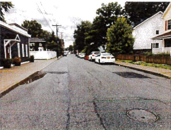
Eliza Street facing south
