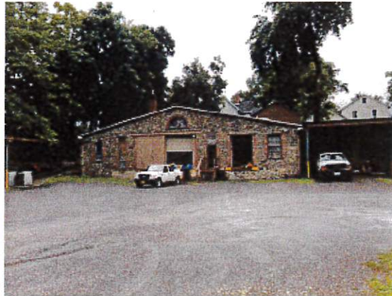
Warehouse front view
