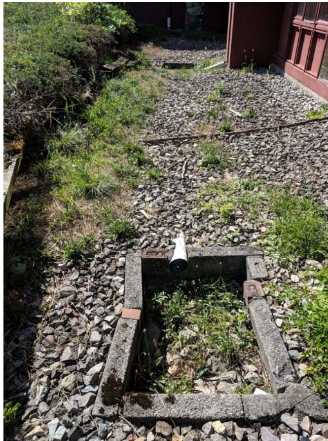
View looking west at the two stone drywells on the south side of the newer addition
