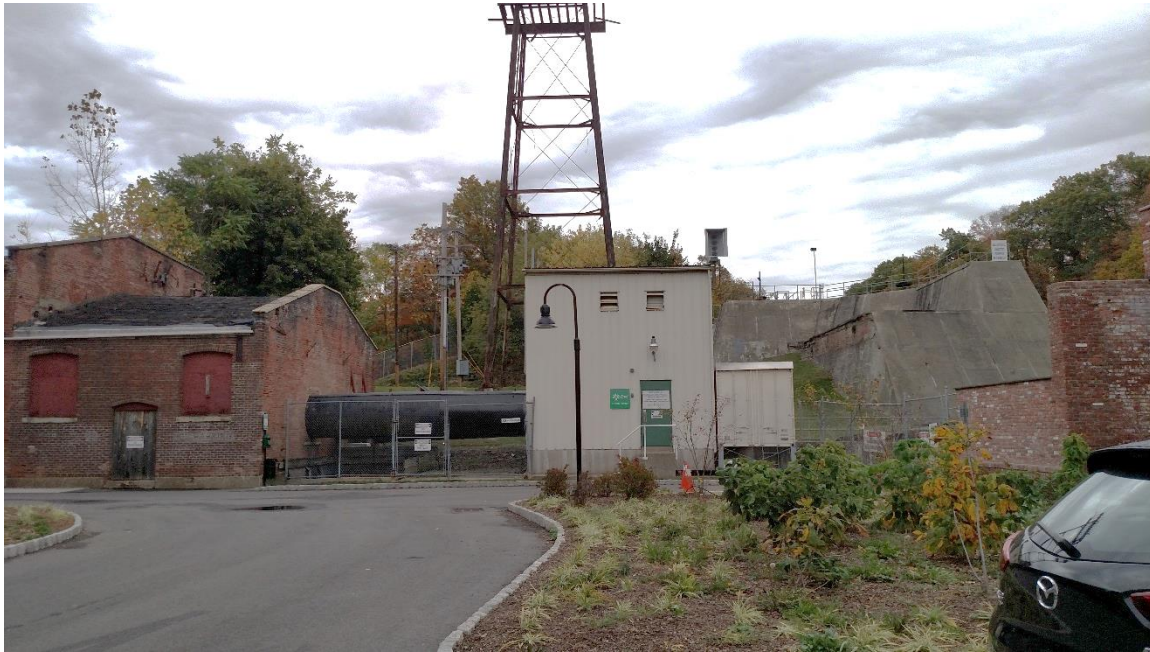
Photo 7: View to the north of the hydroelectric facilities located adjacent to the Groveville Mill Dam. These structures are located to the northeast of the proposed site plan amendment area.
