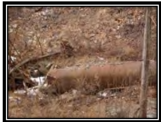
Old Water Drainage Pipe
