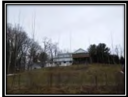
Across Subject Property - Tioronda Ave
