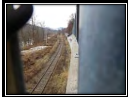
South View of Railroad Line
