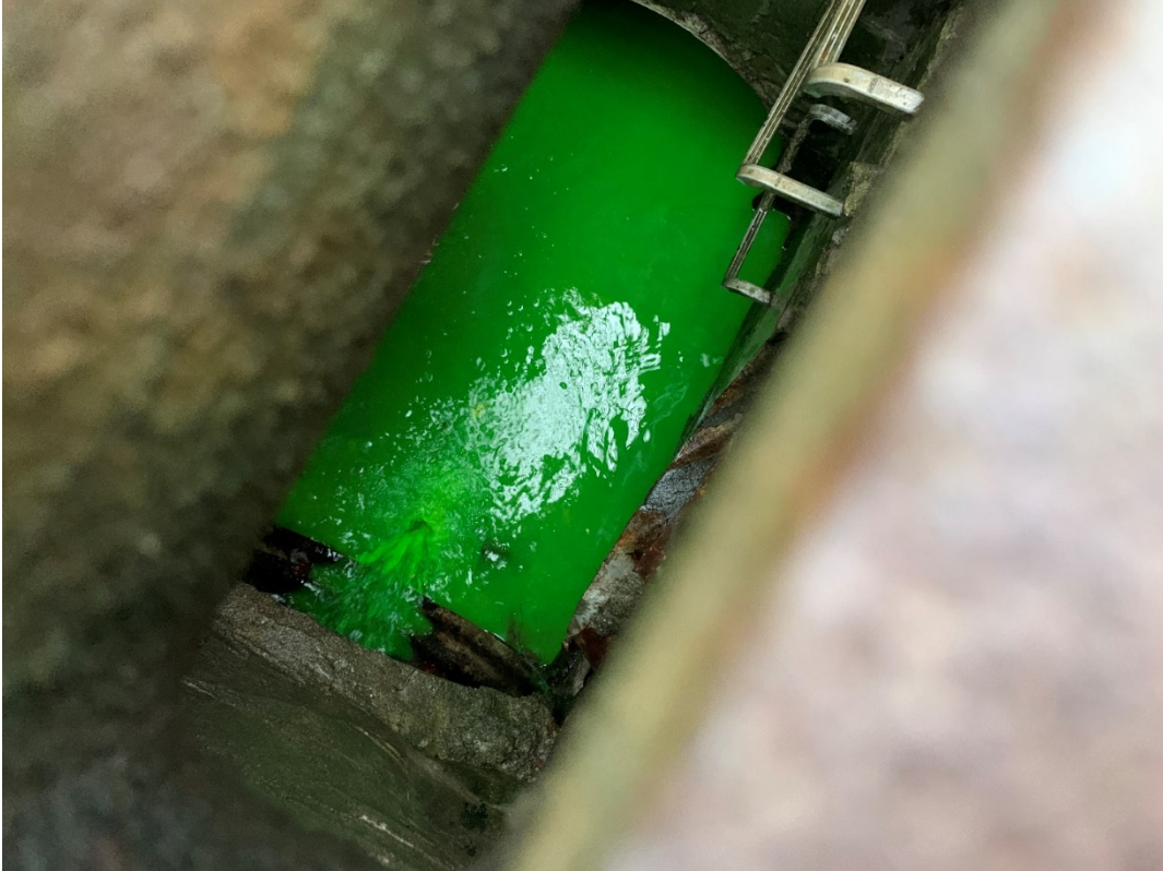
Photo 9: Close-Up of Dye Observed in Bank Street Downgrade Storm Curb Inlet
