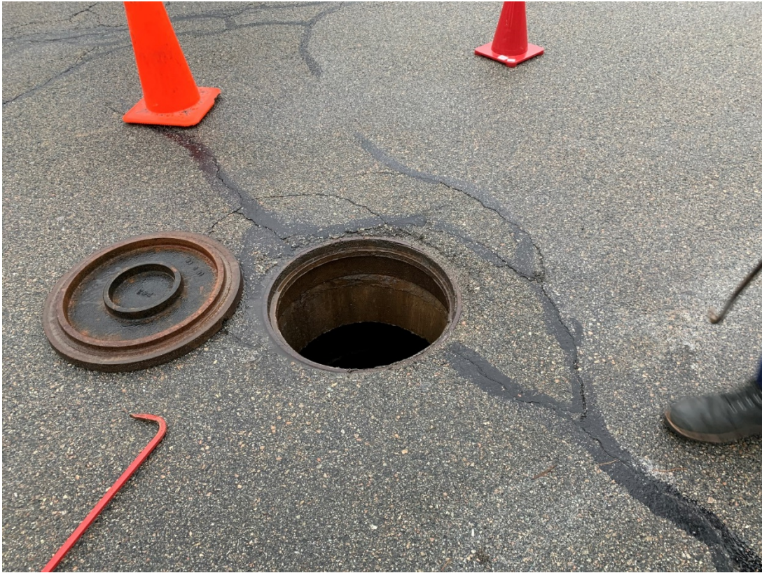
Photo 10: Location of West Main Street Storm Drain Manhole
