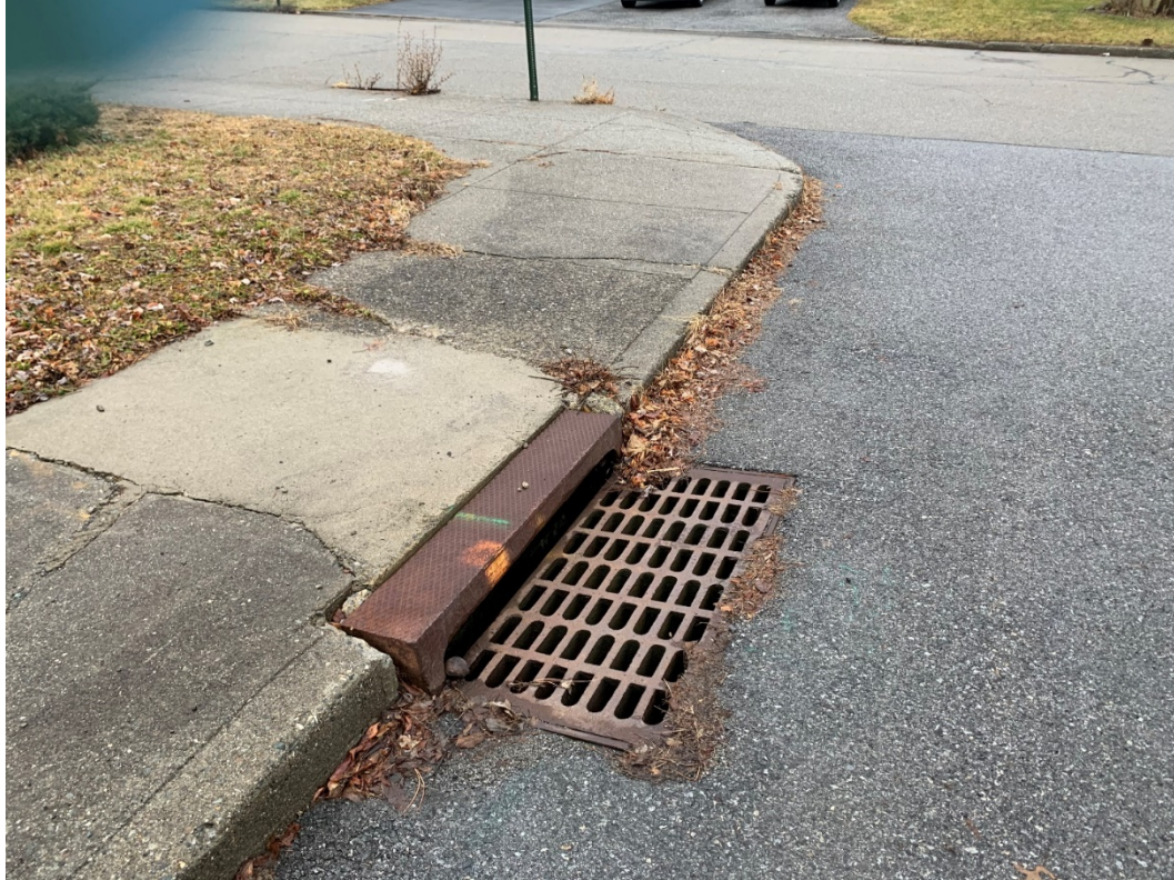
Photo 7: Location of Bank Street Downgrade Storm Curb Inlet
