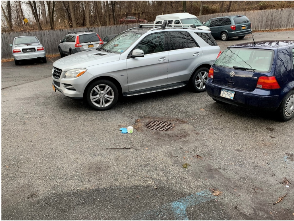
Photo 3: Location of Rear Storm Drain Inlet
