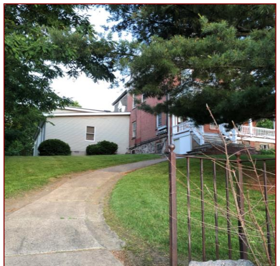
Addition on North Side
