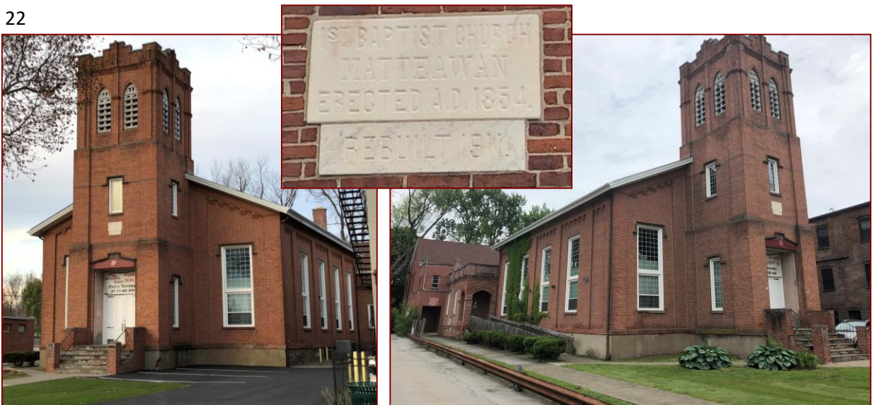
372 Main Street Front View and East Side
