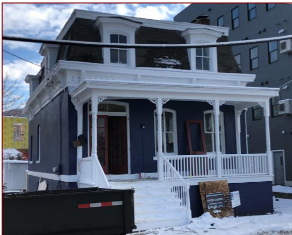
4 North Elm Street
