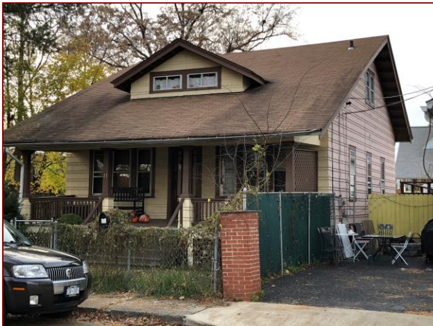
11 North Elm Street
