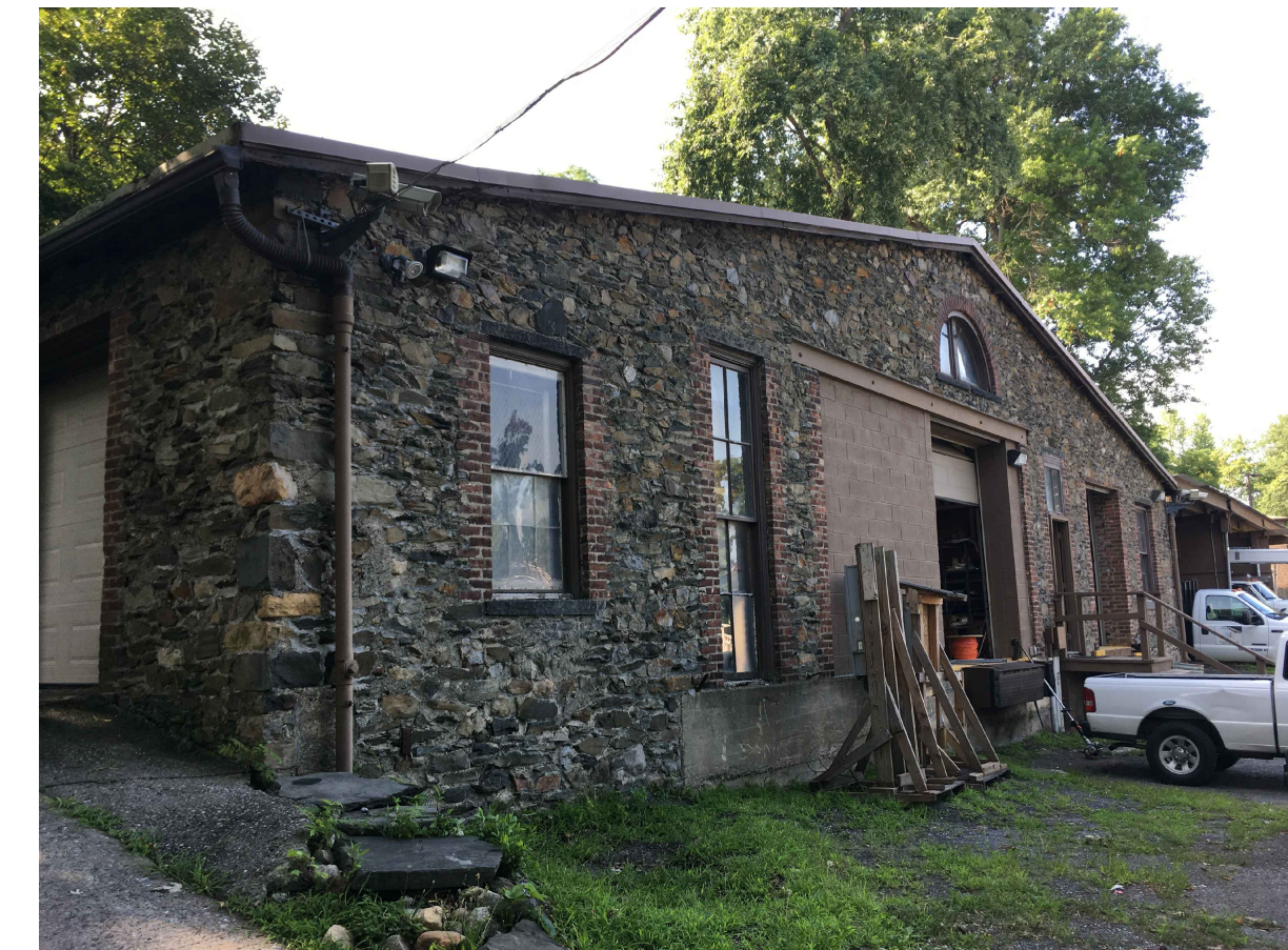
Photo of Existing Stone Building
