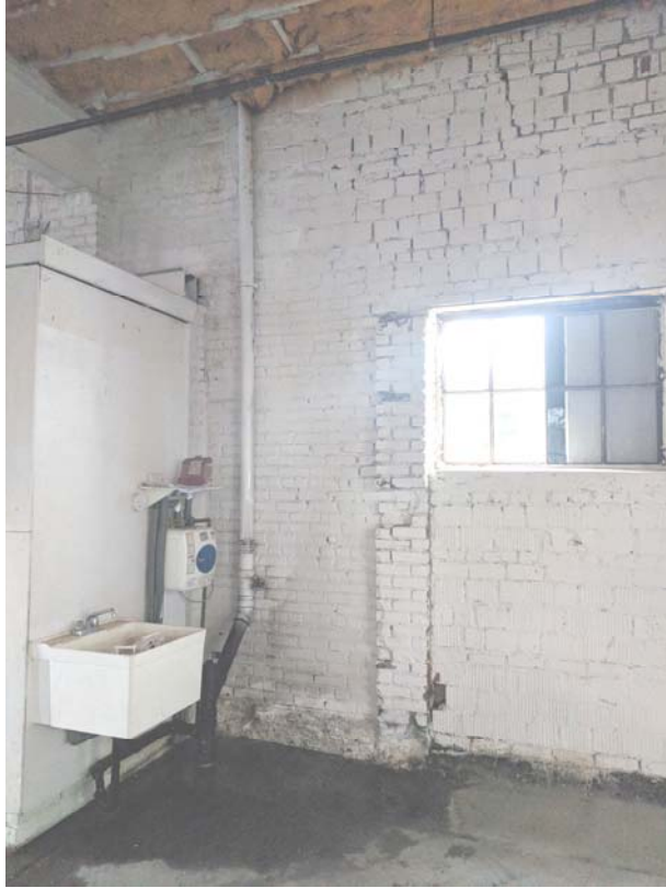
Figure 3 - View of Roof Leader on South Side of Rear Building
