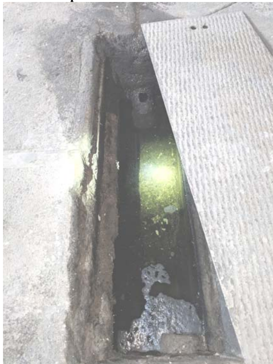
Figure 2 - View of Sump Within Floor of Rear Building
